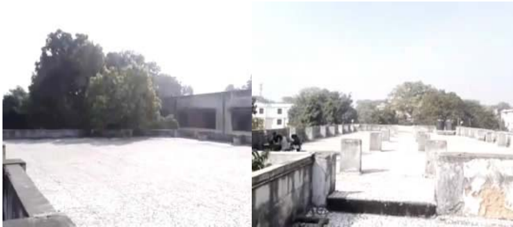
Figure 1: Roof top Picture of the NP Girls Middle School
